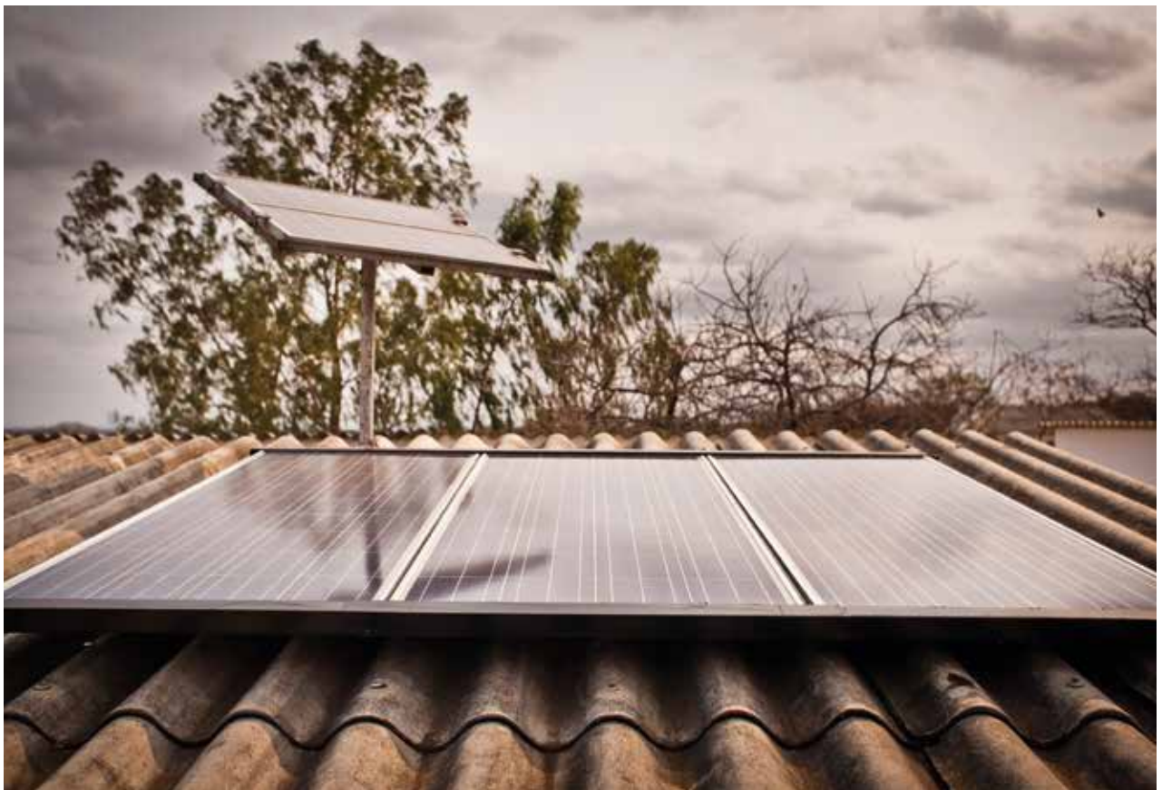
Solar home systems (SHS) offer a cost-effective mode of supplying amenity power for lighting and appliances to remote off-grid households.
