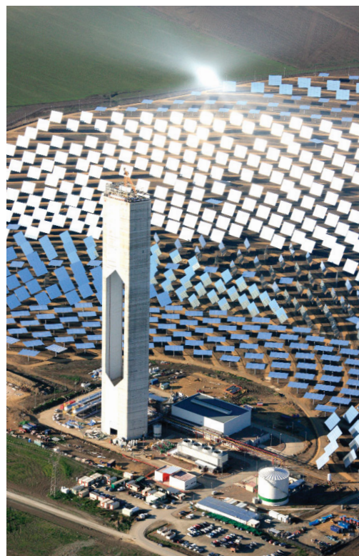
Credit: Abengoa. Powerful, efficient and cost-effective Concentrating Solar Power (CSP) systems work by concentrating sunlight with mirrors to create heat which may be used to raise steam to drive turbines and generators. Heat may be stored in melted salts or other substances so that that electricity may be generated at night or on cloudy days.
